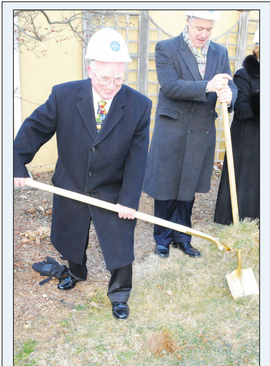
Middleburg Library Advisory Board President Denis Cotter takes the first shovel of dirt at the groundbreaking for an expansion of the facility.
